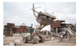
The facility was constructed with a steel frame and masonry exterior. Concrete slabs and foundations were removed and final site restoration was performed.
